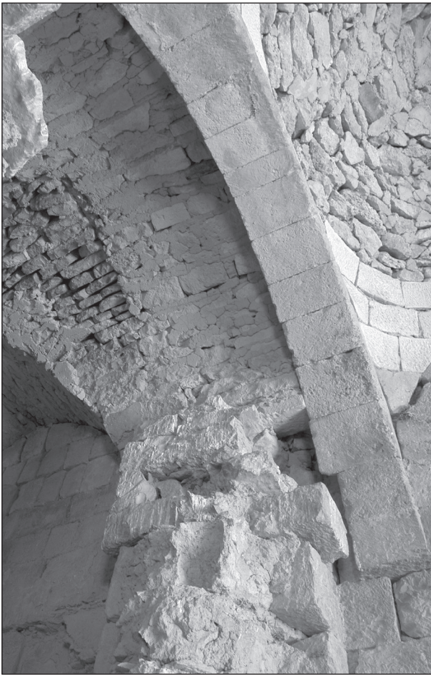
4. Hammām as-Sarāḥ. Internal view of the building after the restoration. Note the reconstruction of the dome, and the northern arm of the tepidarium's cross vault, erroneously elongated in the 1974 restoration till the southern arch of the dome's pendentives. This area was originally occupied by the "venturi suction chamber", opened to the sky.
