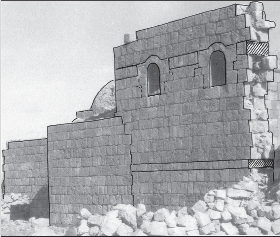
9. Ḥammām as-Sarāḥ. Construction phases: Detail of the joint between the frigidarium (to the left) and the audience hall (to the right) abutting on the former. Note the distinctive change of building technique in both stages (Cropped photo from DoA Archives).
