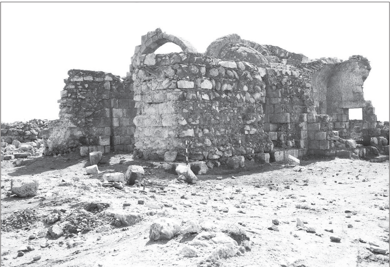
3. Hammām as-Sarāḥ. View of the building in 1974 before the DoA intervention. DoA Archive.
