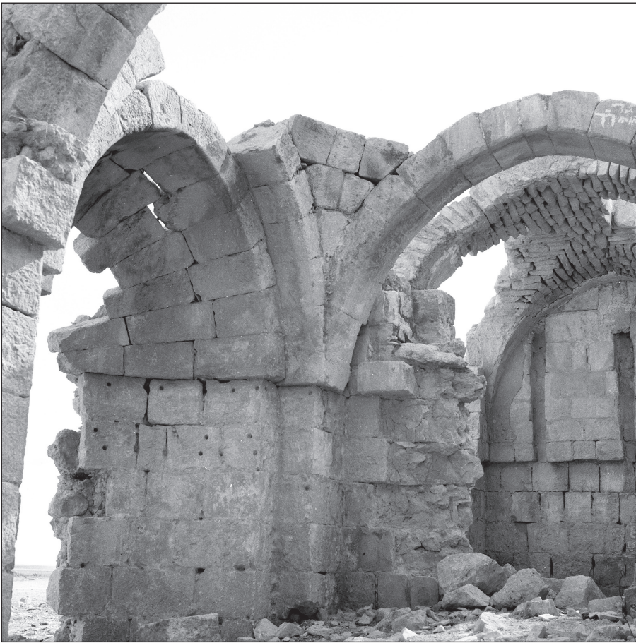
6. Ḥammām as-Sarāḥ. Internal view of the building before the restoration. Note the remains of the lateral semi-domed recesses, the pendentives, and the tepidarium 's cross vault in the background. DoA Archive.
